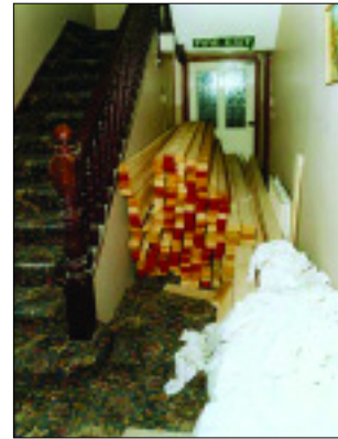
Figure 9: A blocked corridor with incorrect signage
