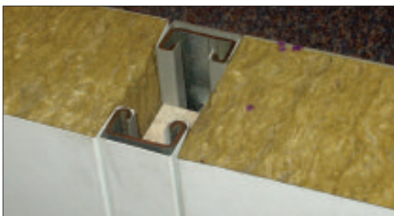
Figure 17: Insulated core panel – internal
