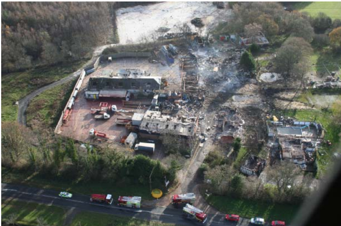
Photograph of site taken on Monday 4 December 2006
