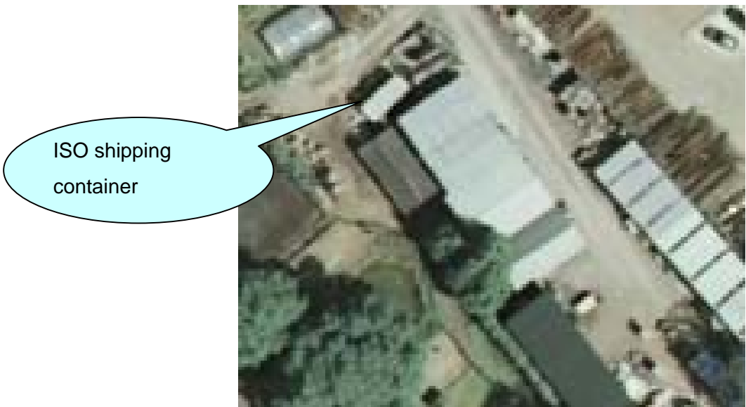
Photo showing location of ISO container
